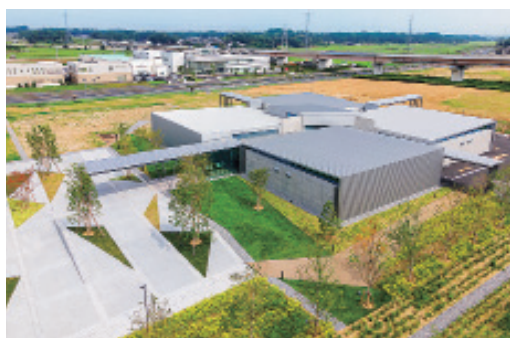
Photo 4: Exterior view of the RISO R&D Center II facility.
